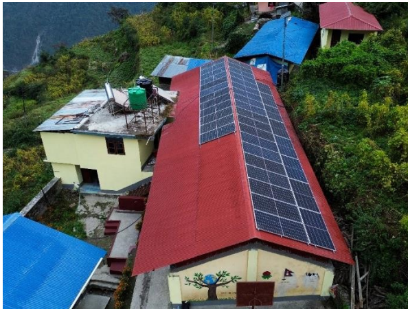
Figure 14: Completed PV system on the roof, 21.3 kWp
